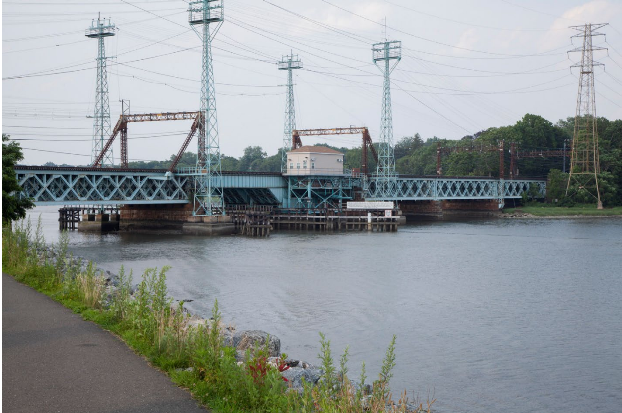
Figure 3-8. Cos Cob Bridge
