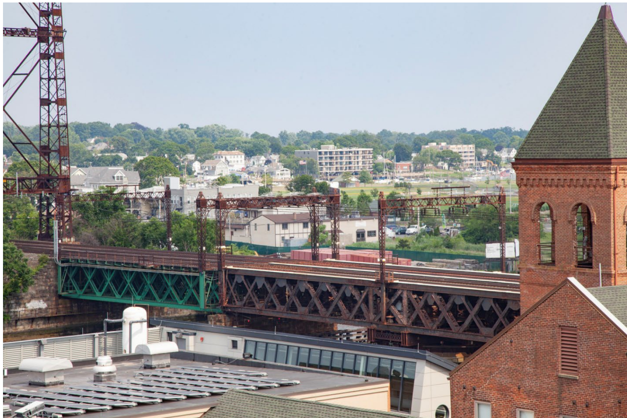
Figure 5-3. Walk Bridge in Norwalk, Connecticut
