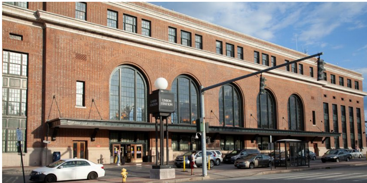
Figure 2-14. New Haven Union Station
