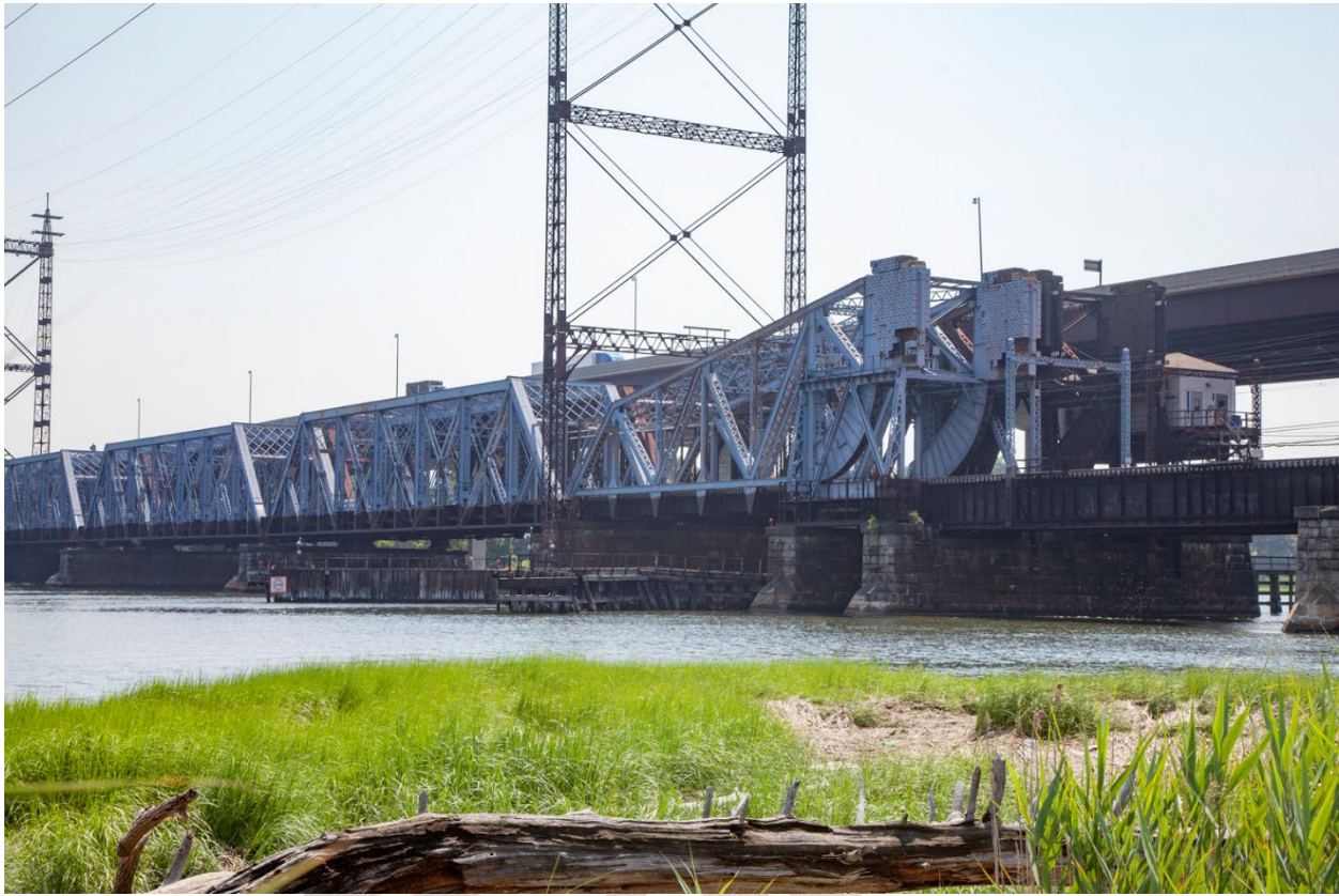
Figure 3-9. Existing Devon Bridge
