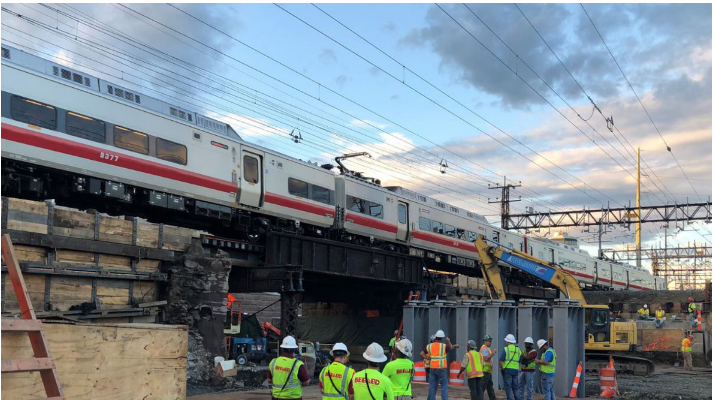
Stamford construction site
