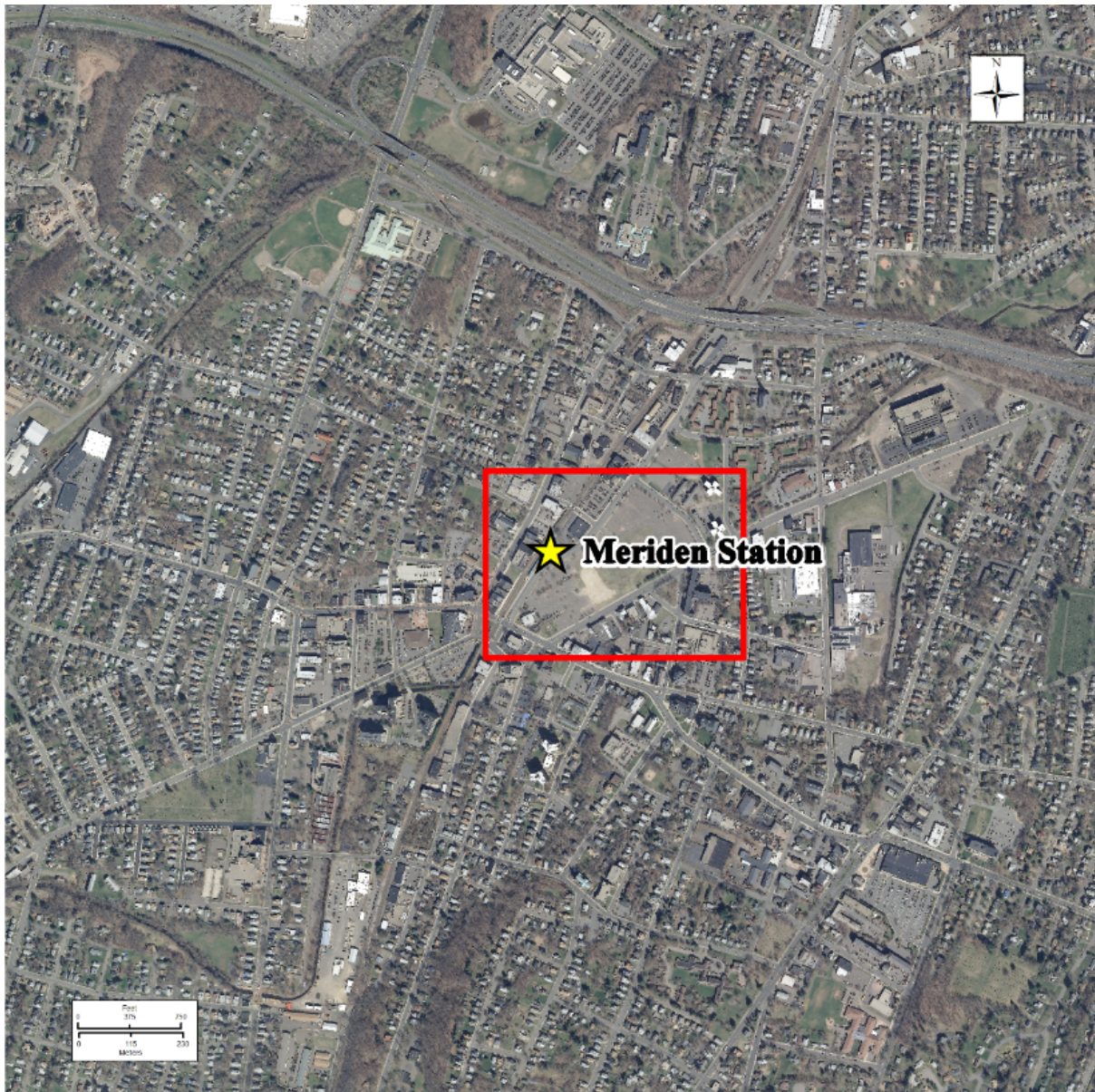
Figure 22. Aerial View of the Hartford Line Station in Meriden, 2011 (source: DEEP)
